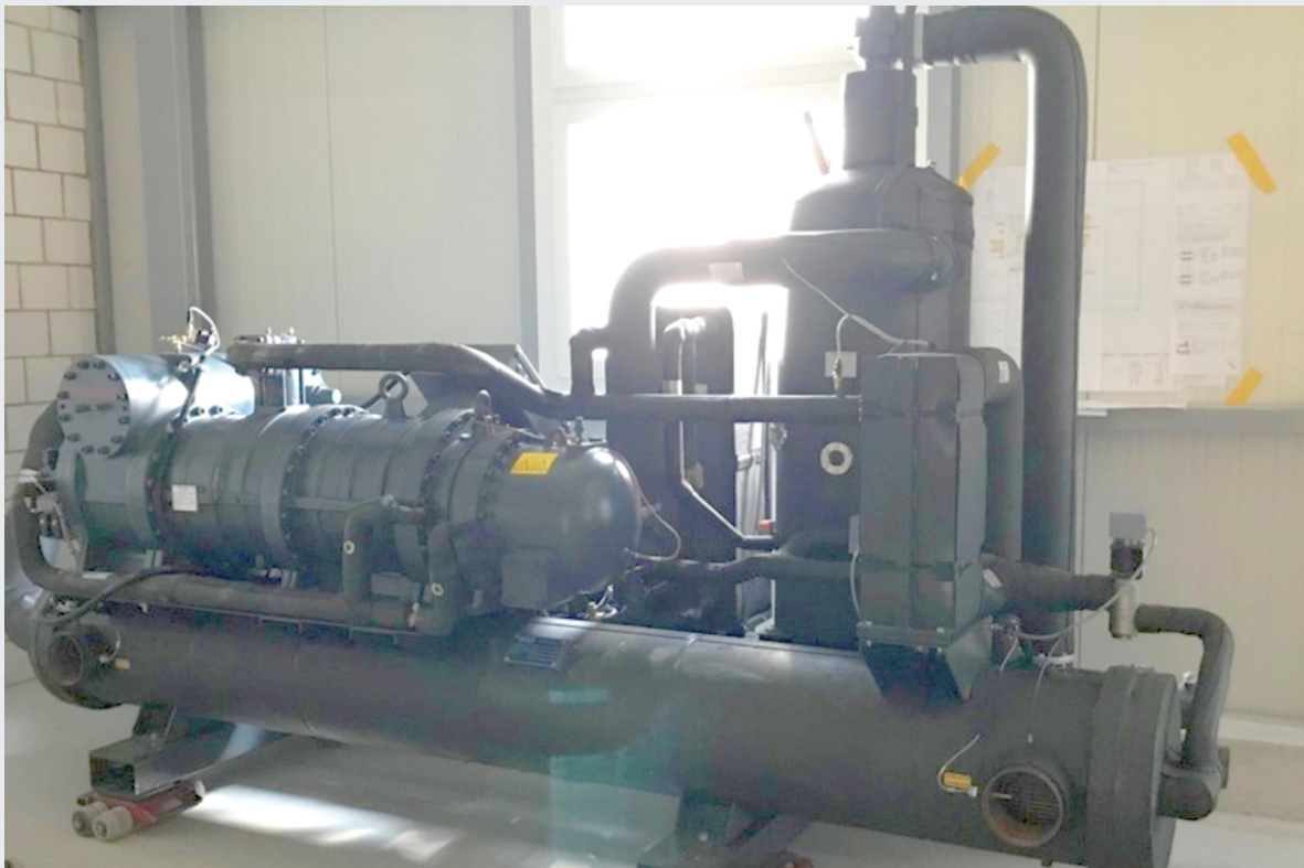
Fig. 1: From Waste Heat to Cheese [3]. Data centre (Rechenzentrum Ostschweiz) built by the St. Gallisch-Appenzellische Kraftwerke AG in Gais Appenzell [1] feeds the waste heat into a district heating network. The mountain cheese factory uses this waste heat as a heat source in a high temperature heat pump to generate process heat for cheese production.
