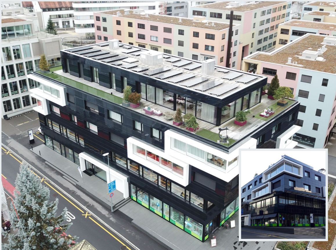
Fig. 1: Different views of the monitored building Black & White in Switzerland, with mixed residential and office use.
