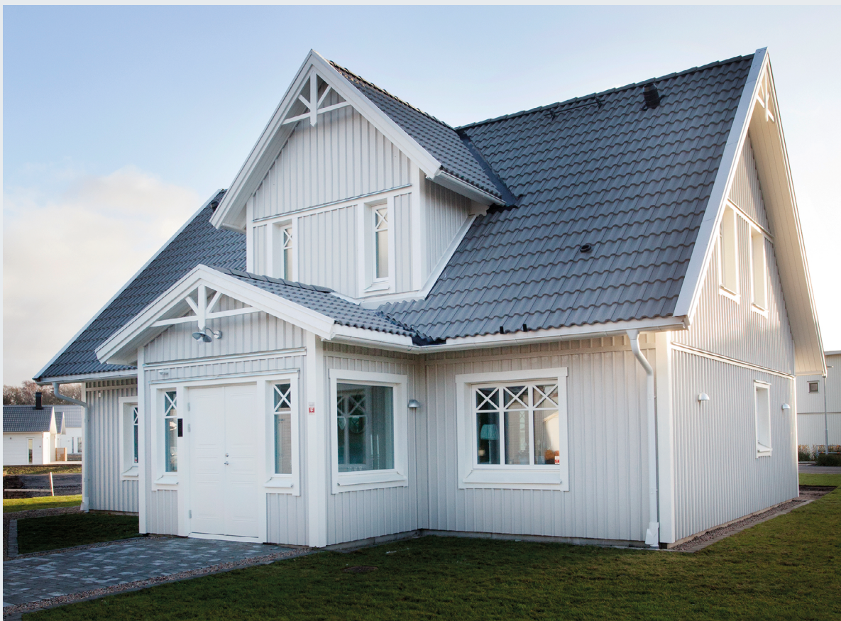
Fig. 1: Twin houses in Sweden used for the evaluation of different heating system characteristics and the evaluation of different heat pump control.
