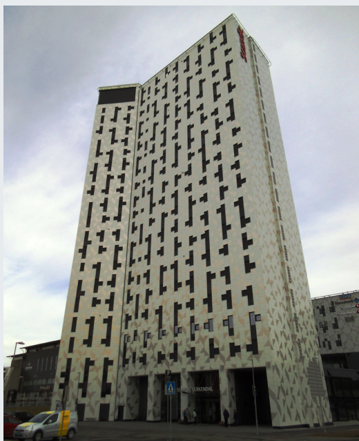
Monitoring project Scandic Hotel in Trondheim
