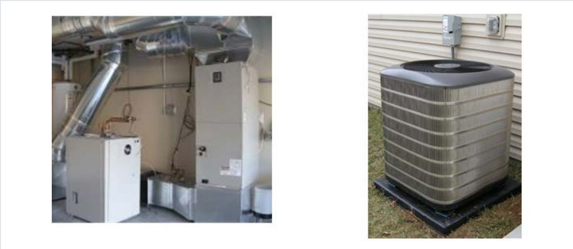
Figure 2. AS-IHP 1 field test prototype installation; left) indoor sections (hot water storage tank, compressor and water heating module, and indoor fan coil), right) outdoor section.
